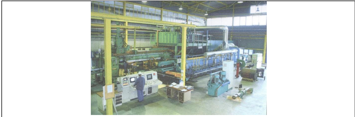
Figure 43: EXALCO extrusion machine installation
